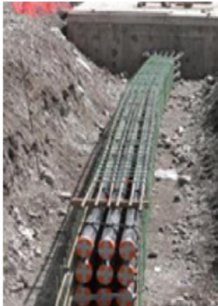
Example of underground conduit for duct being placed in a trench before concrete is poured
