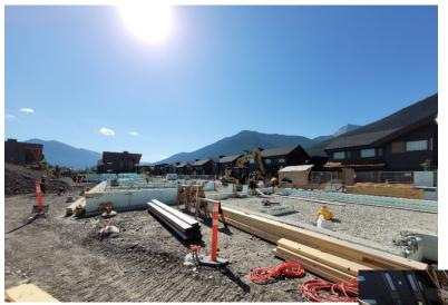
Construction of the south building foundation continues. Another concrete pour has completed the foundation walls for this building. Backfill of the foundation is finished and wood framing can now begin.
