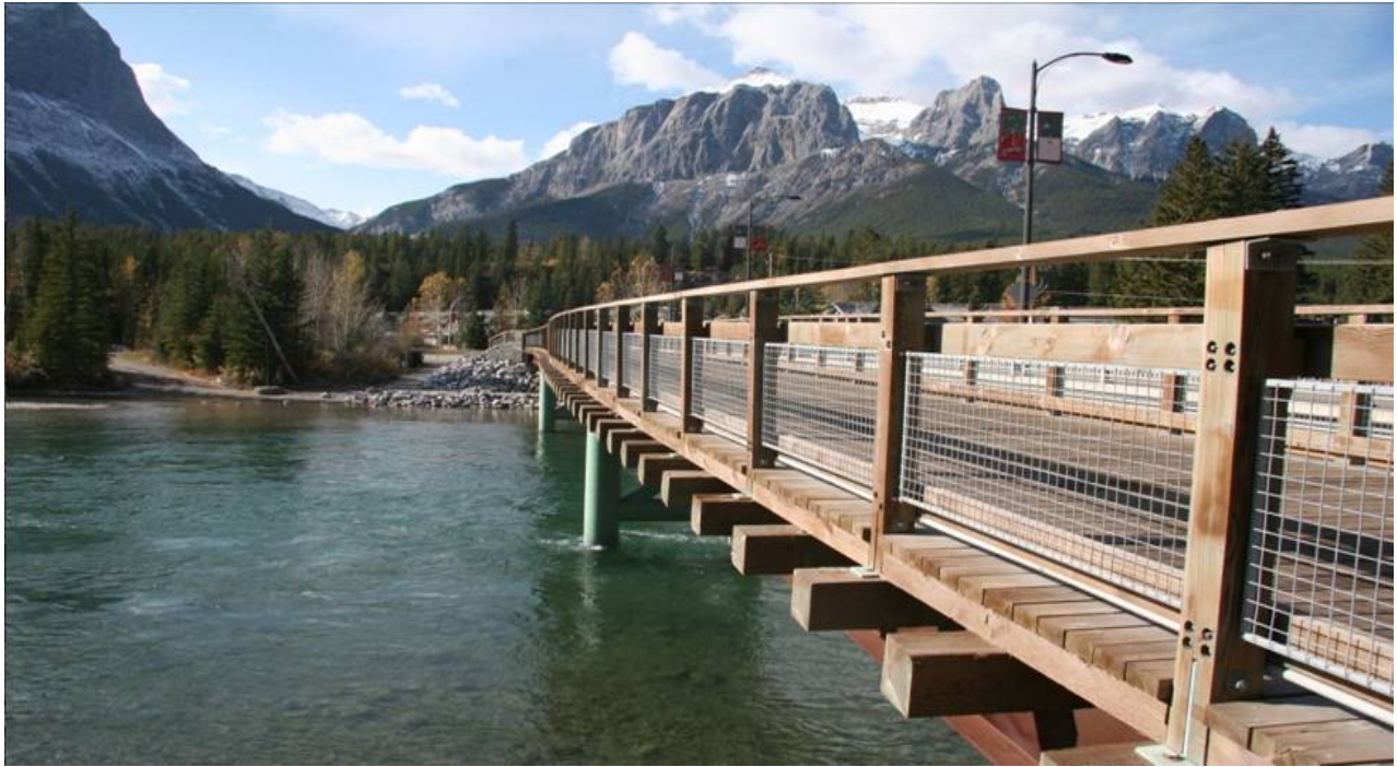
Figure 6: Bow River Bridge
