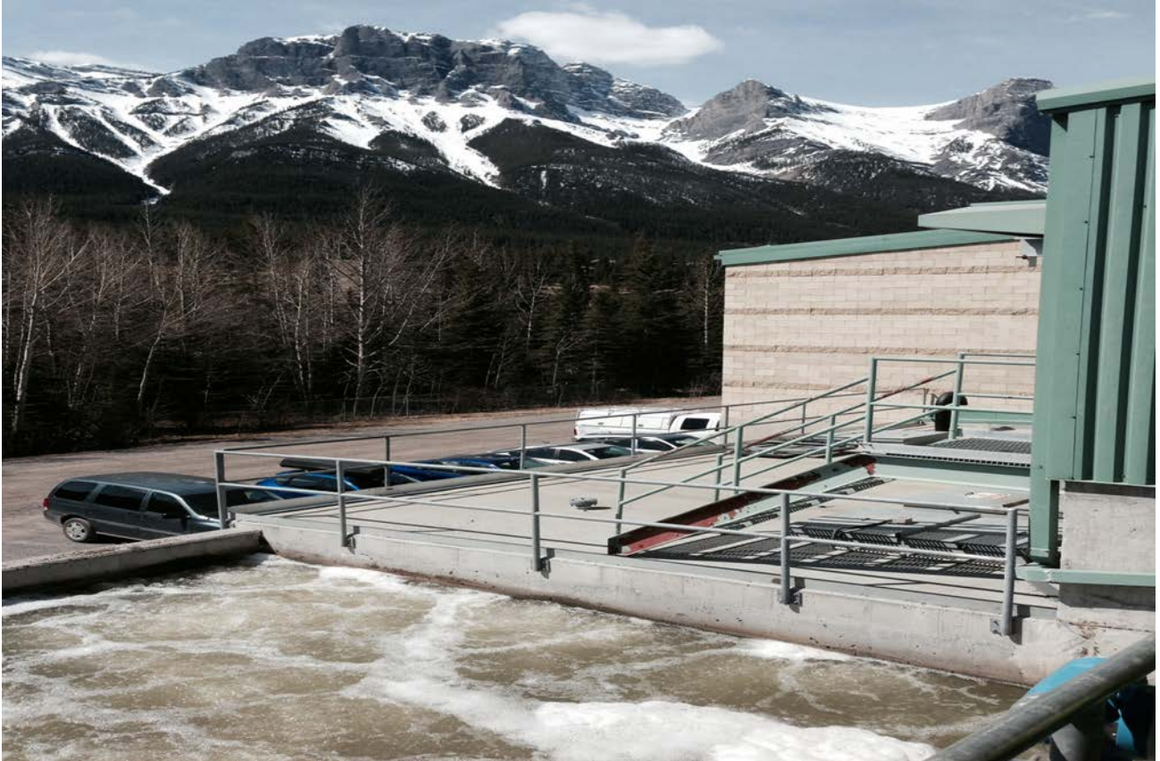
Figure 9: Wastewater Treatment Plant
