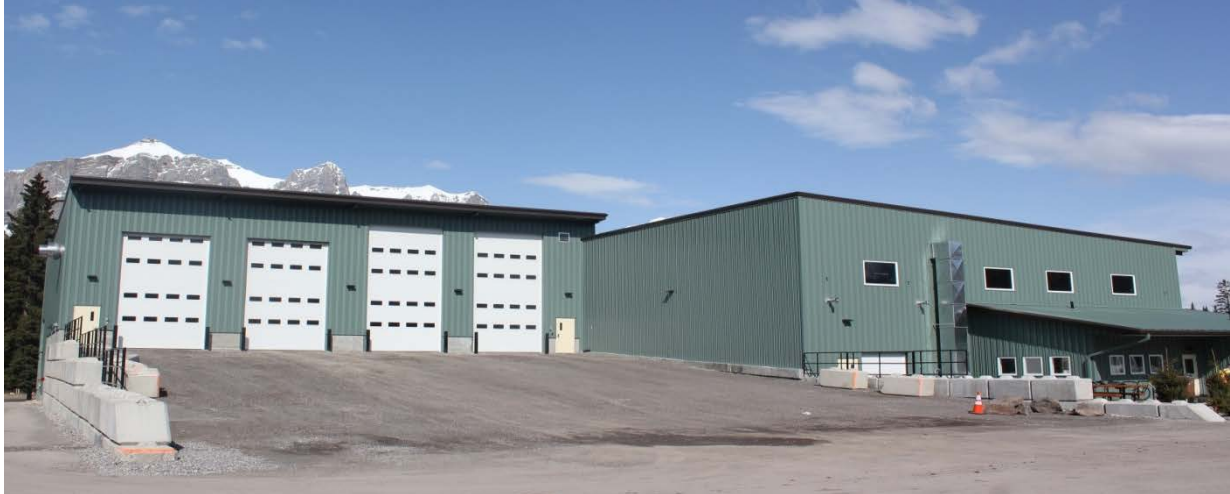
Figure 5: Materials Recycling Facility
